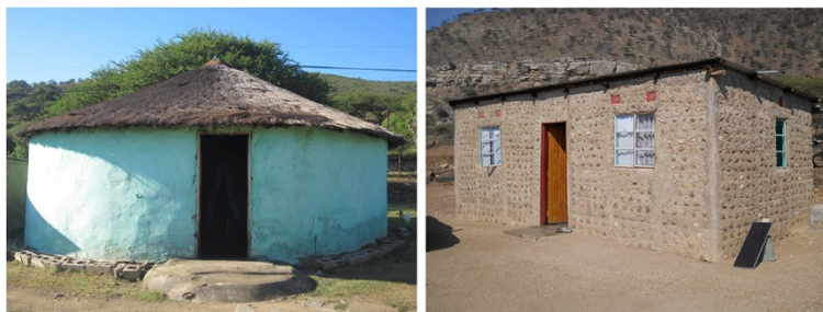
Figure 1 Two predominant types of traditional home construction in Tugela Ferry. A. Round-shaped home with thatched roof B. Box-shaped home with metal roof.
